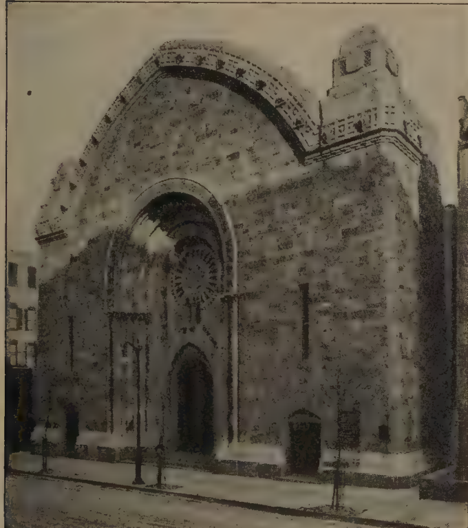
798 Walter S. Schneider, architect; Henry B. Herts, associated; photograph by Wurts Brothers
